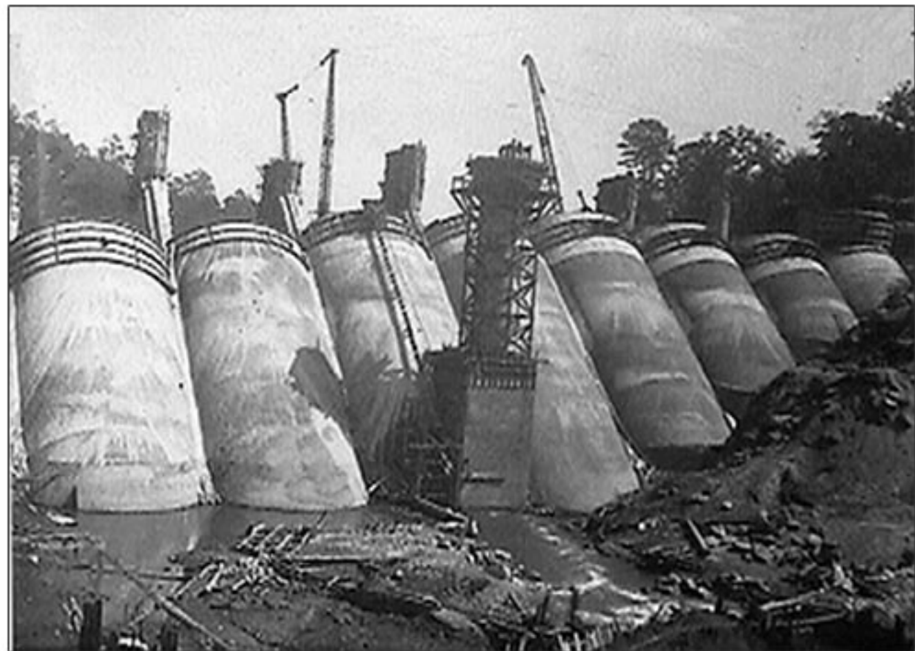
The Lake Lure dam under construction
